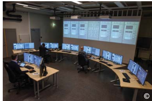
Fig. 1. Layout of the multi-unit SMR control room simulator and operator workstations.
