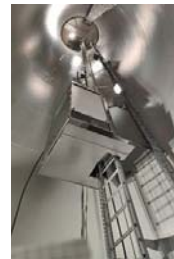
Figure 2. Lift inside turbine
