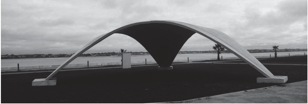
Fig. 1 – Full scale prototype of the double curved concrete shell.
