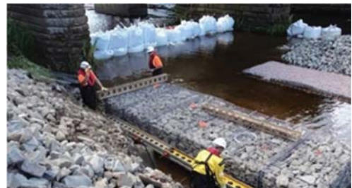
Figure 1. Scour repair works of the case study bridge, reproduced from Tola et al. (2025).
