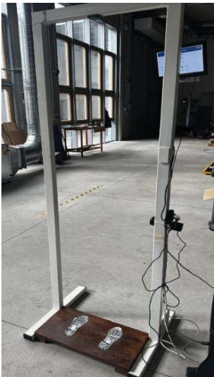
Fig. 4. Final installation of the smart gate in an industrial environment, showing the complete assembly with structural frame, sensors, display, and operator platform
