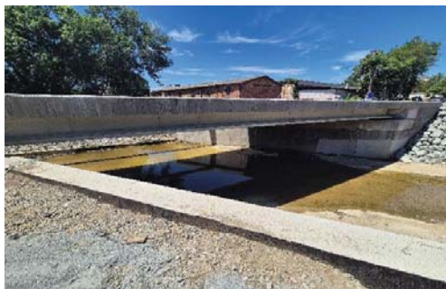
Fig. 7. Bridge – “White shore” – new structure
