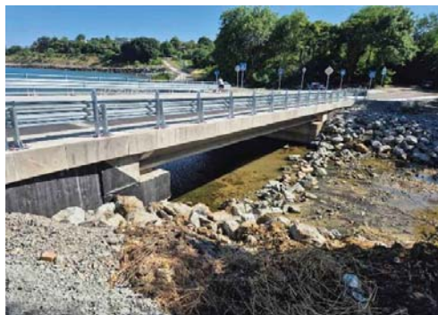
Fig. 9. Bridge – “Coastal Alley” – new structure
