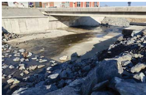
Fig. 8. Bridge – “Mandrata” – new structure
